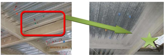
The flutes parallel to the top flange of the beam are required to be fully packed with spray fireproofing to the edge of the beam flange or other approved methods per NFCA Bulletin 1003.
