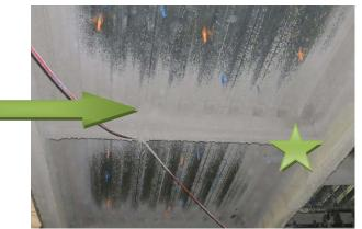
The flutes perpendiular to the top flange of the beam are required to be fully packed with spray fireproofing to the edge of the beam flange or other approved methods per NFCA Bulletin 1003.
